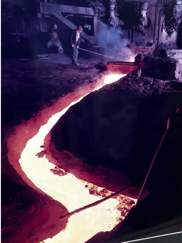
Tapping Blast Furnaces - FT Industrial Photographer of the Year 1969
